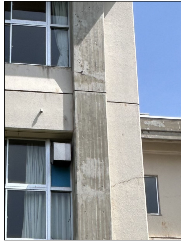
補修箇所②
